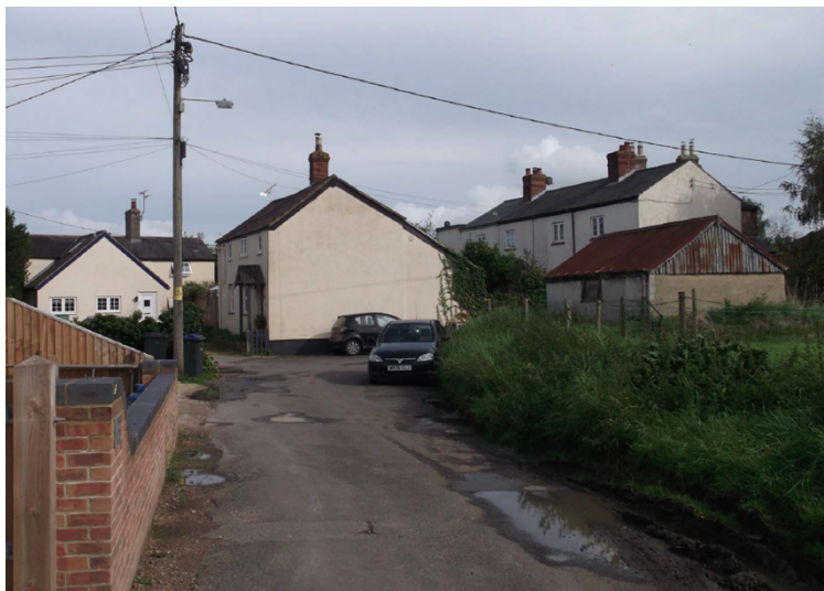
Photo of existing outbuilding to be removed and the existing embankment between Bunnies Lane and the site
