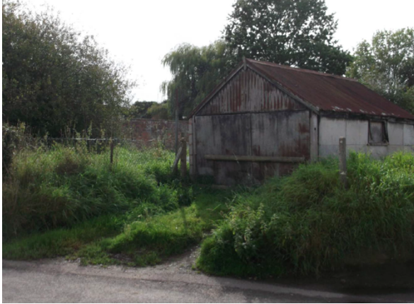
Existing access onto Bunnies Lane from existing outbuilding on site
